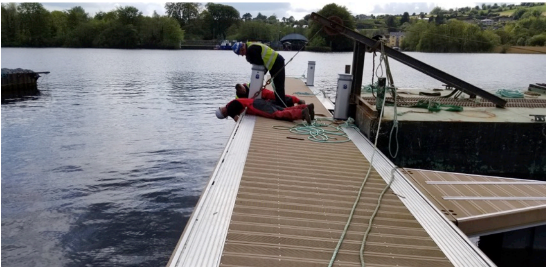
Tensioning using a winch
